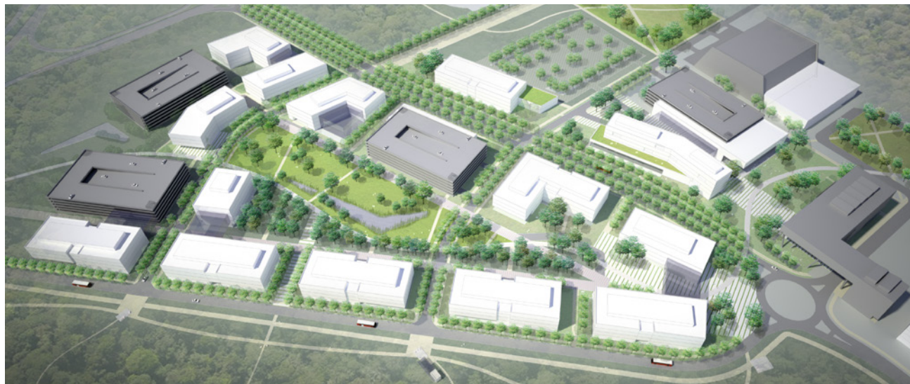
Figure 1.13 View of high-tech research and innovation park
