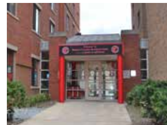
ID64 Panel applied to canopy
